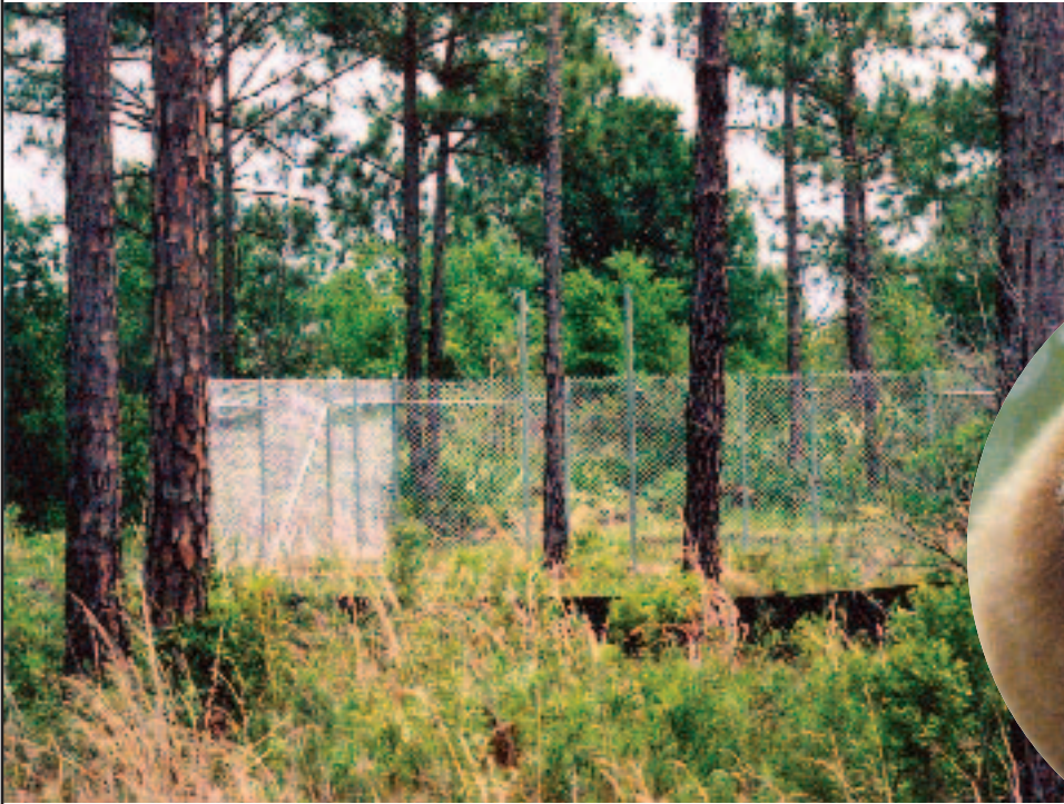
▲ The perimeter fence erected around the yet-to-be-constructed quarantine shelter.
