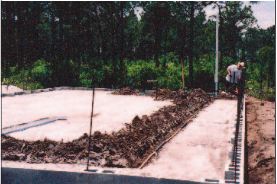
▲ Plumber working on the foundation of the new lemur shelter.
